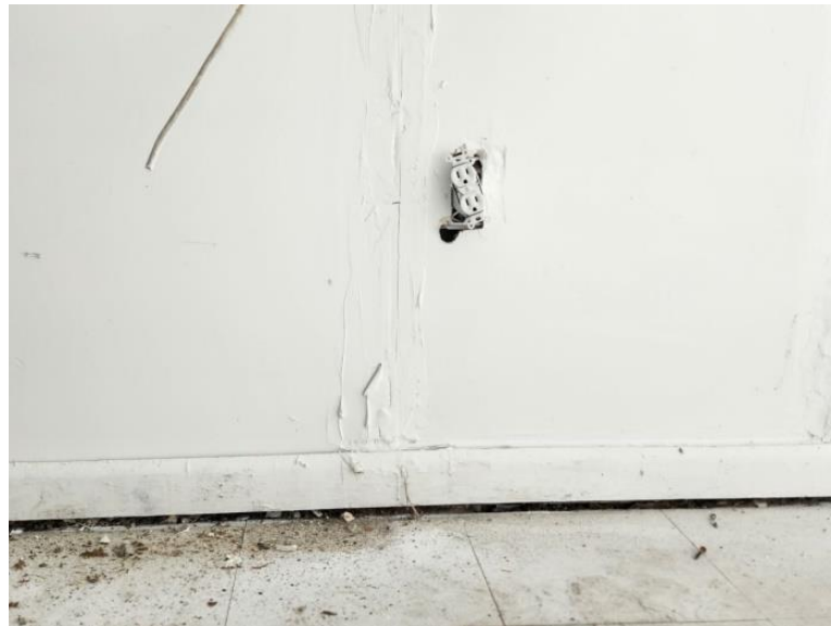
Figure 1; Close up of unfinished-room details. Located in Apt #110 room 2
