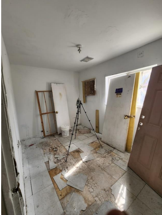
Figure 4; Apartment #110 room 1, taken during receiving measurements for STC test
